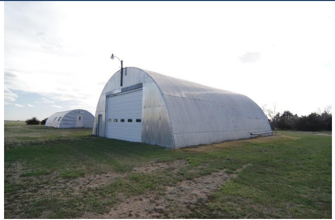
Quonset® type building of 2000 sf
