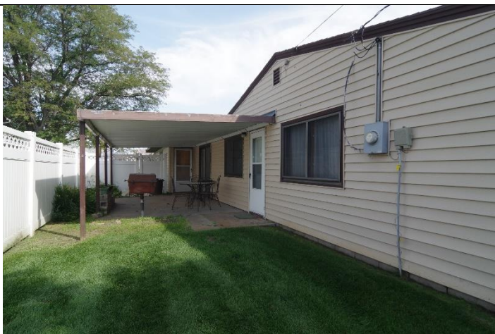
Covered patio on north side of home with gas grill
